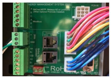
Peer to Peer and BMS use RJ45 Ethernet cable in one of the plugs on PCB06 and plug the other end into the next boiler (no hard wiring to lugs)
