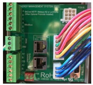
Peer to Peer and BMS use RJ45 Ethernet cable in one of the plugs on PCB06 and plug the other end into the next boiler (no hard wiring to lugs)
